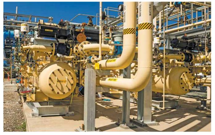
In 2012, this gas compressor unit was one of two installed at Bulwer Island. The units provide for any reduction in pressure of natural gas to the BP Oil Refinery which the Bulwer Island Co-generation Station serves.
