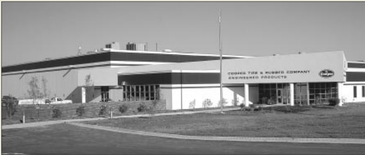
In July Cooper began producing extruded rubber hose and hose assemblies at its new manufacturing facility in Mt. Sterling, Kentucky. Construction began on the 178,000-square-foot plant in late 1995 and was completed in mid-summer 1996—on budget and on time.
