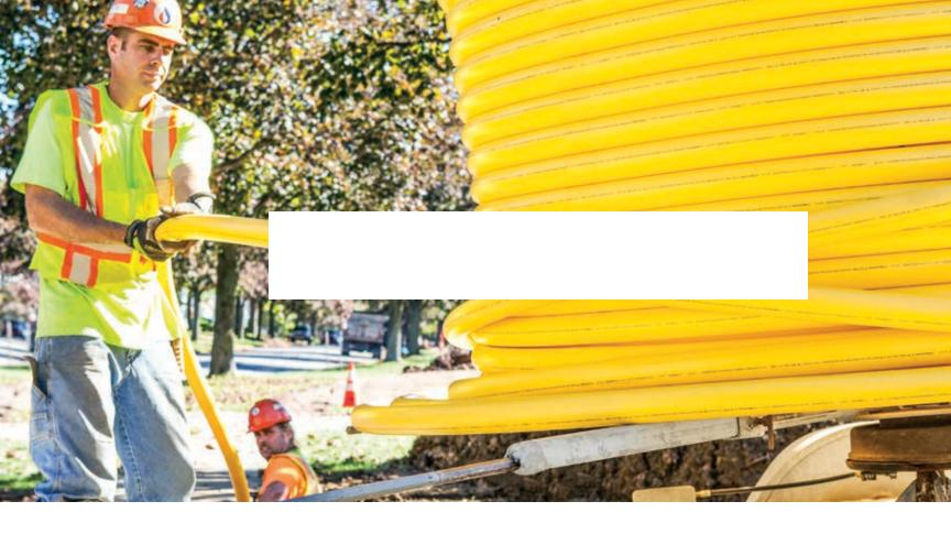
Above – The Utility continues to modernize its steel and cast iron infrastructure. Here, Utility employees Wiley Tothill and Sean Bannach undertake a routine insertion job in which plastic pipe is inserted into the existing steel pipe, minimizing excavation damage.
