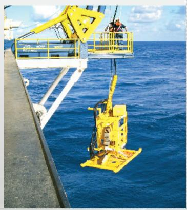
INSTALLATION WORKOVER CONTROL SYSTEM (IWOCS) DEPLOYMENT
