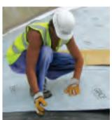
substrate from deteriorating, building designers chose Grace Prepufe® 300 R waterproofing membrane, applied below the slab to stop water migration around the substructure. Bituthene® 8000 HC waterproofing membrane protected the substructure walls from the harsh
