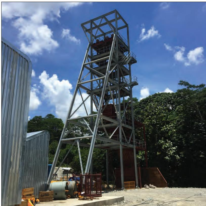
Picture 3: E15 Head Frame at 80% completion
