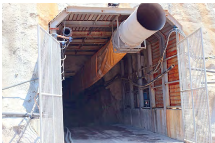
Portal to Main Access Decline
