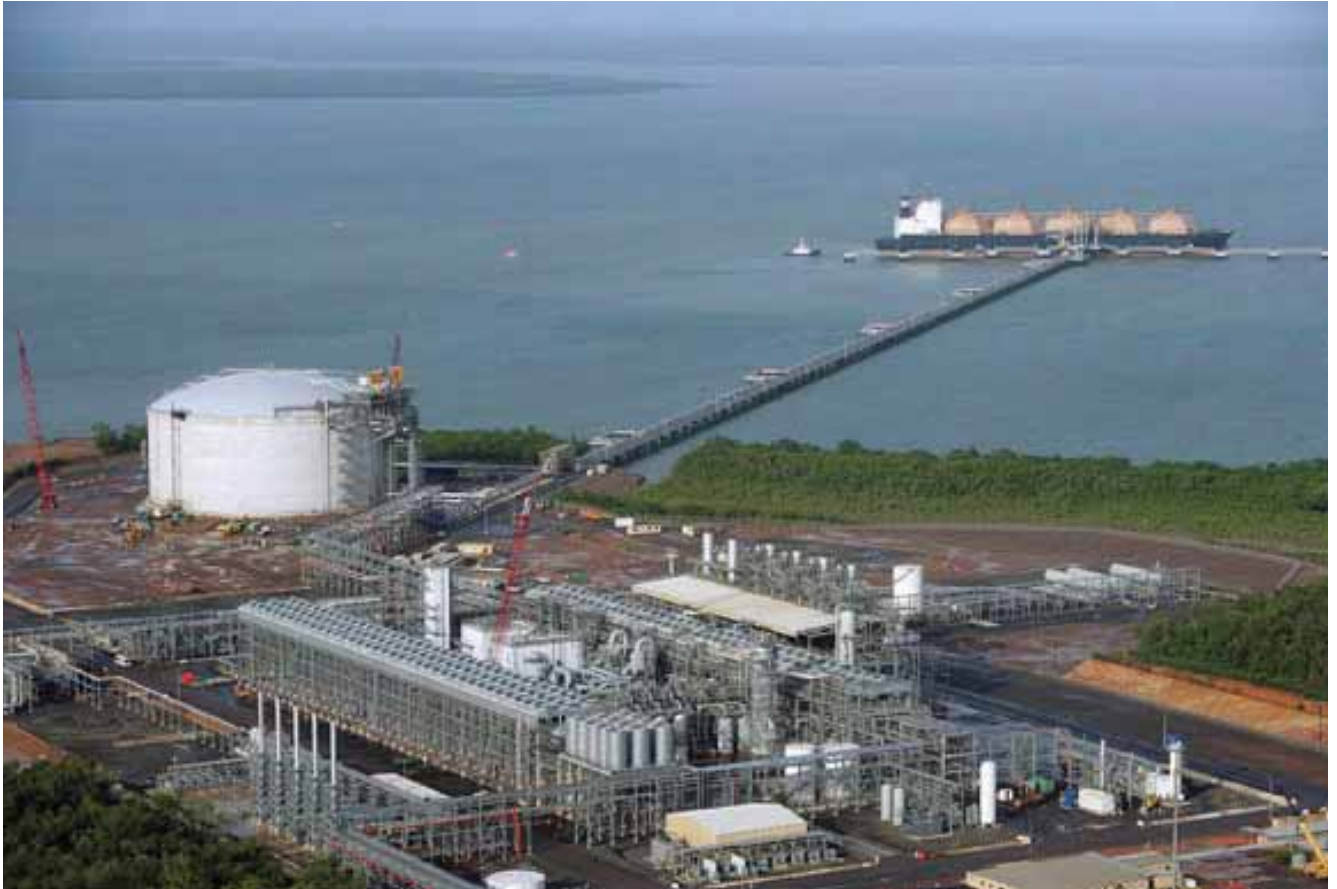
Darwin LNG processing and load-out facility.
