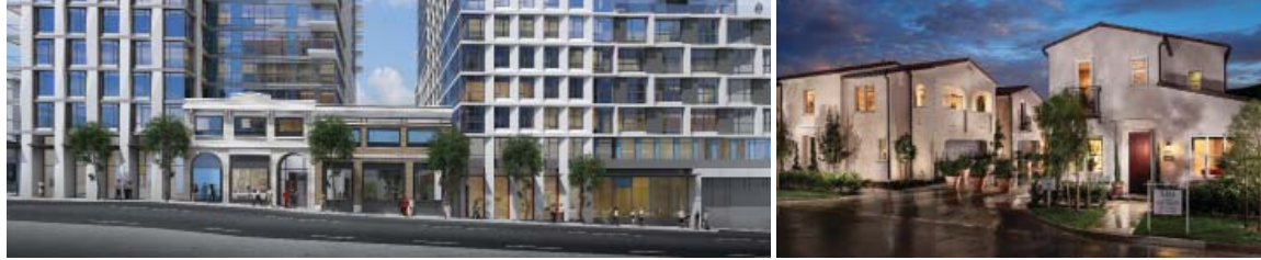
Above, left to right: Rockwell, San Francisco, California (THP1 US); and Villa Metro, Santa Clarita, California (THP2 US)
