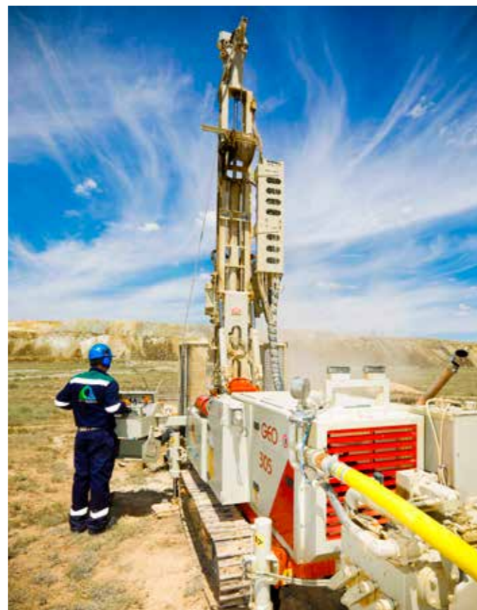
Drilling boreholes at Kounrad
