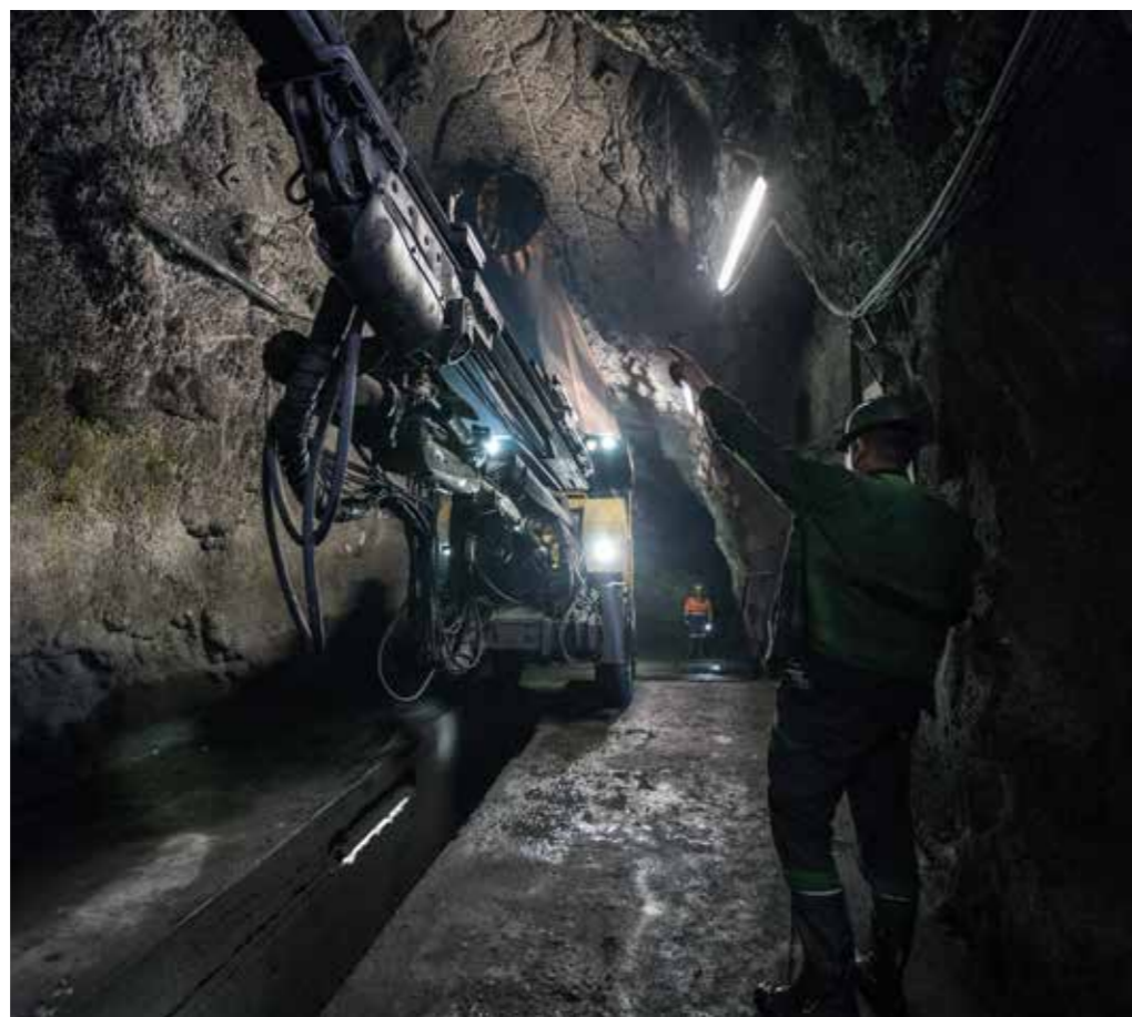
Drilling at Sasa
