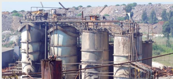
South African gold recovery processing plant
