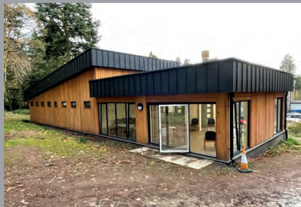
The visitor changing and washroom facility at Wiston Lodge
