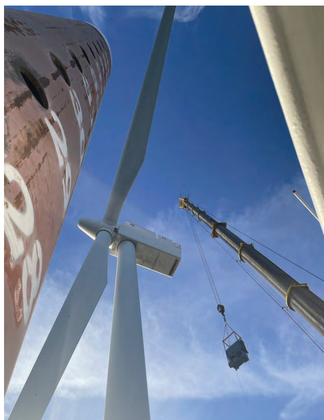
Rhyl Flats generator exchange
