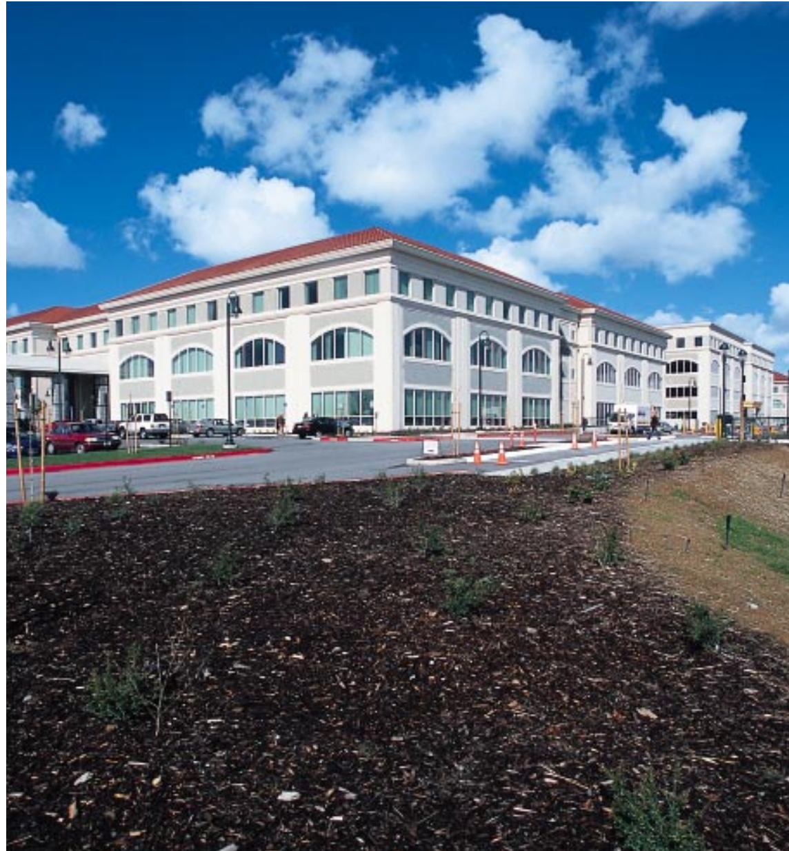
Granite Regional Park in Sacramento is a former Granite quarry that has been converted into a revenue-producing office park as well as a public park in a creative partnership between Granite, the City of Sacramento, and a developer.
