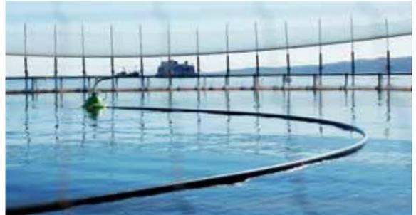
The final piece of infrastructure was commissioned in 2H2020, the transfer pipe, taking fish directly from the nursery to the wellboat. This transfer method eliminates the use of truck transfers, and improves fish health and performance following the transfer from freshwater to seawater, as the fish are less stressed.
