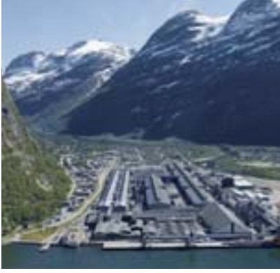
The expansion of our Sunndal plant in Norway has established a new industry standard for aluminium smelter technology.
