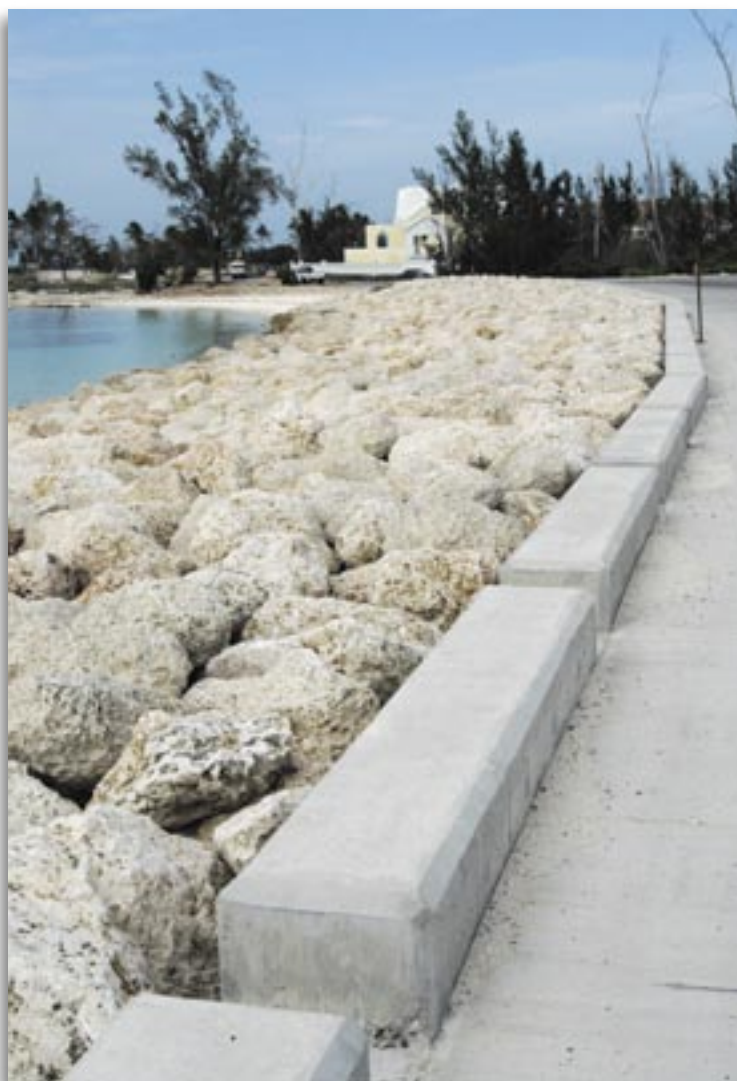
BAHAMAS • Hurricane damage to a sea wall in Nassau was repaired under the Immediate Response Facility for Natural Disasters and Other Emergencies.
