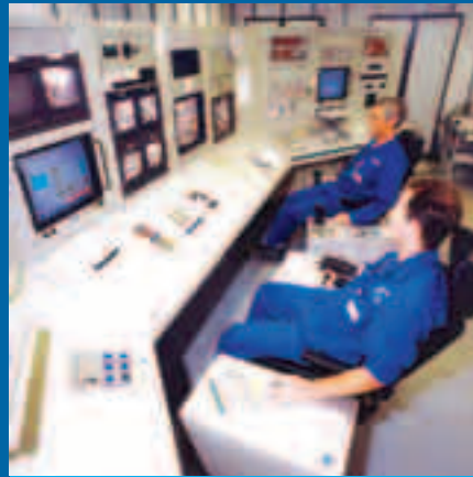
JF Nuclear decommissioning control panel
