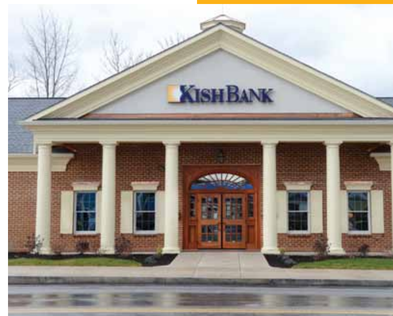
The new McVeytown Branch
