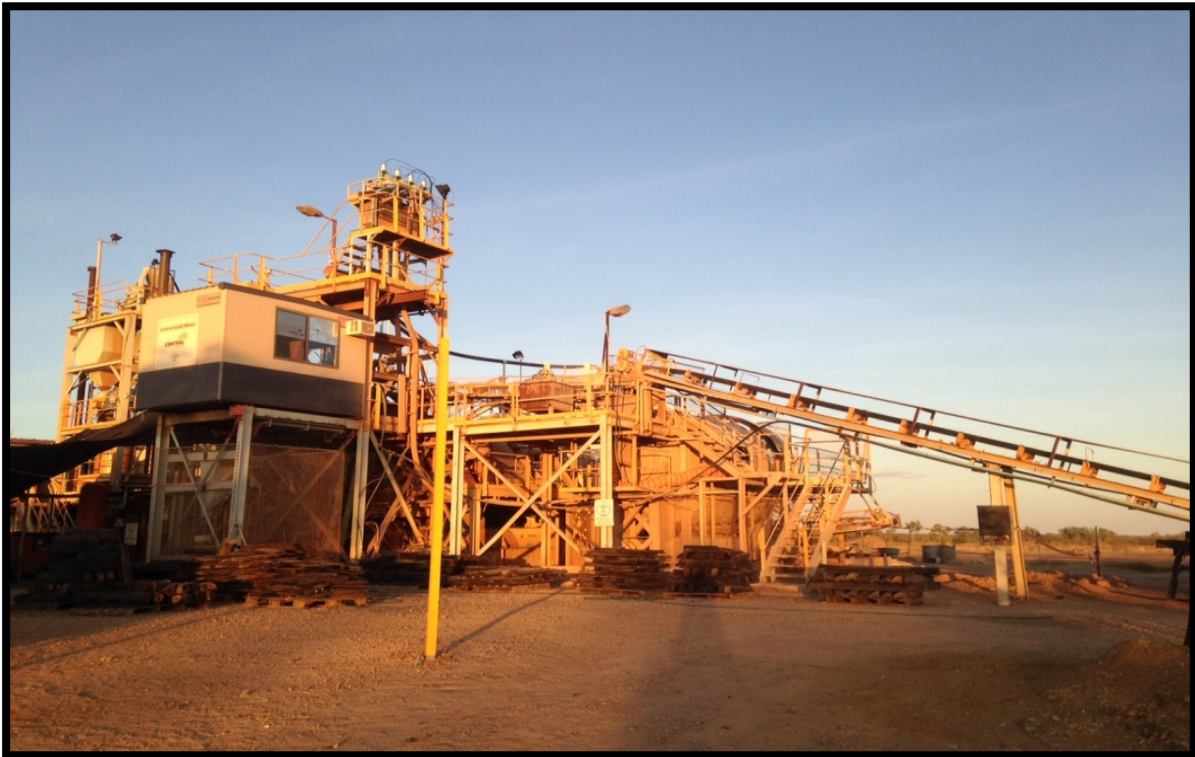
EOPL's Georgetown Gold Processing Plant
