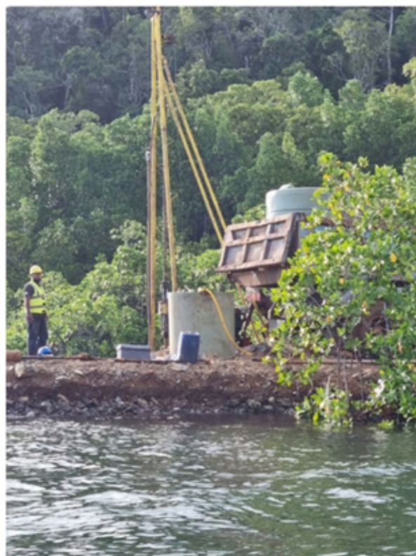
Figure 4 – Geotechnical Drilling for Wharf Construction
