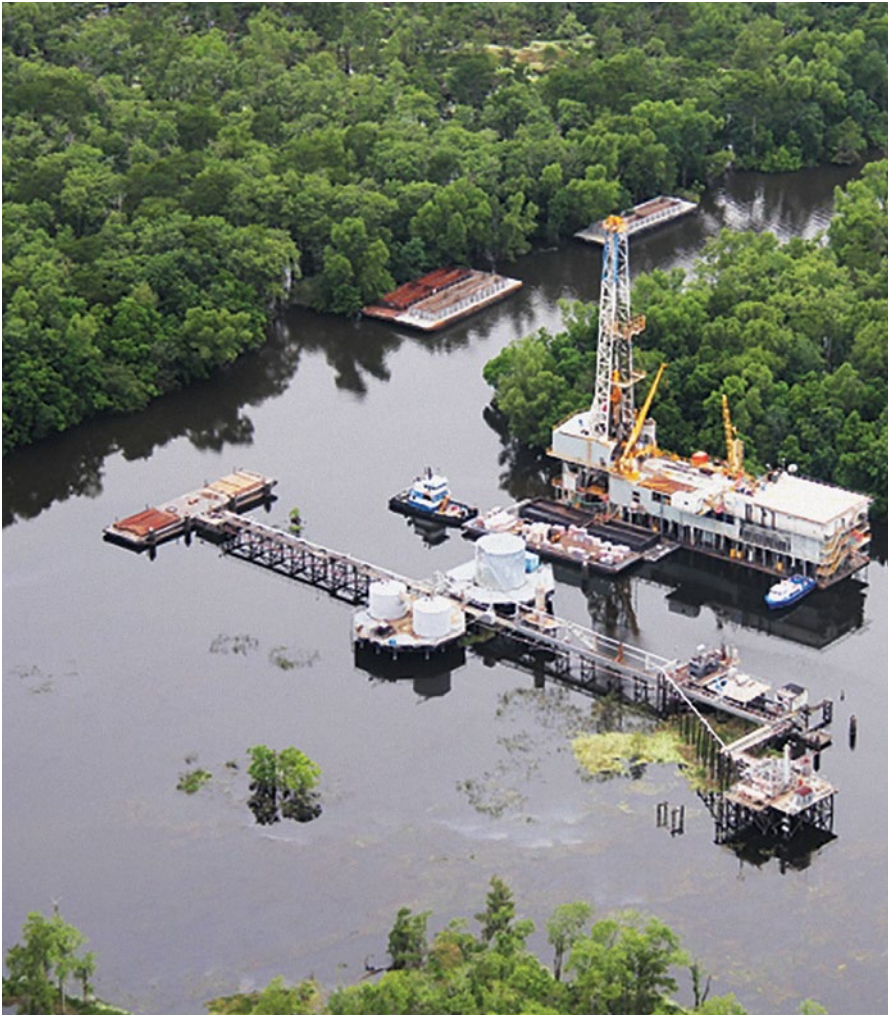
Right: Williams No.2 Alt. discovery well – Barge drill rig next to production & oil storage facilities.
