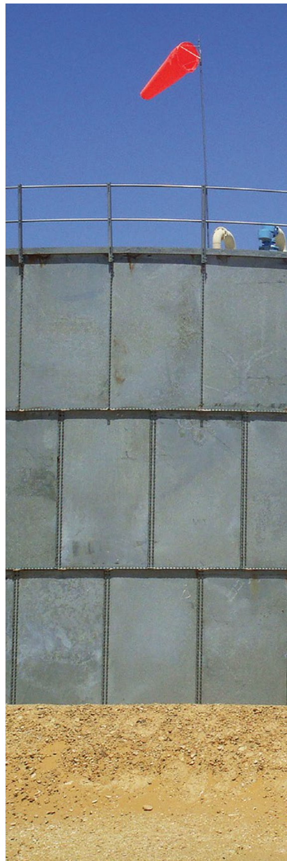
Damis (Block S-1) Yemen – An Nagyah Oilfield: Production and storage facilities.
