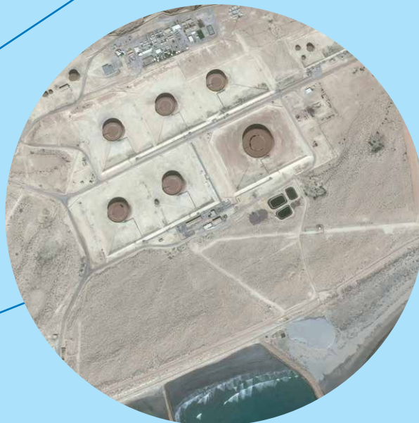
Above: Ash Shihr Oil Terminal aerial view
