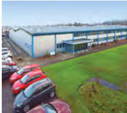
Wardpark Industrial Estate, Cumbernauld
