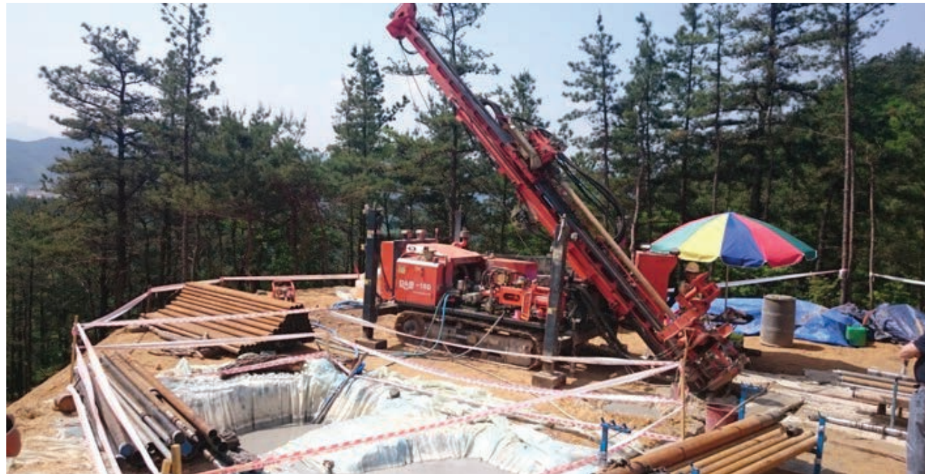
Diamond drilling at the Weolyu Au-Ag Project, South Korea
