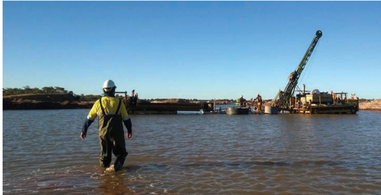
Diamond drilling at the Glandore Gold Project adjacent to the lake margin.
