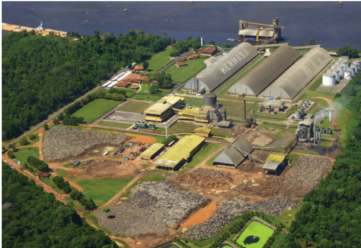
Brazil Potash – Logistics facilities near Manaus
