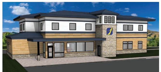
The new Ellsworth branch will be located on Beechland Road.
