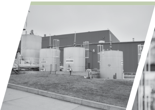
CanmetENERGY pilot facility
